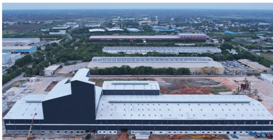
Aerial view of Phase I Quartz Processing Plant
