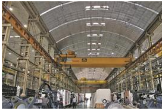
Roof with Overhead Crane
