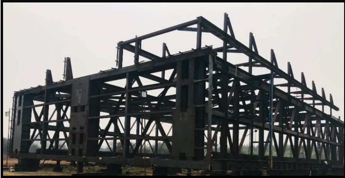
(Accumulator Structure built by us for John Cockerill India Limited)
